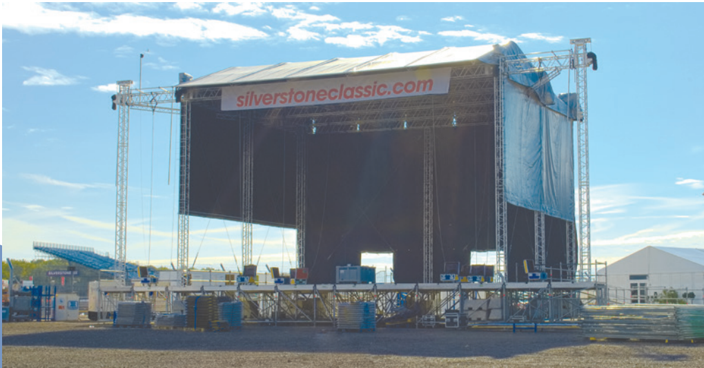
Silverstone Classics, Structure during construction with Concrete Ballast
